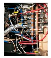
A copper water manifold comes standard, ensuring equal water pressure throughout your home. And each water line is clearly labeled and has its own shut-off valve, allowing you to isolate a single line without shutting off water to the rest of your home.
